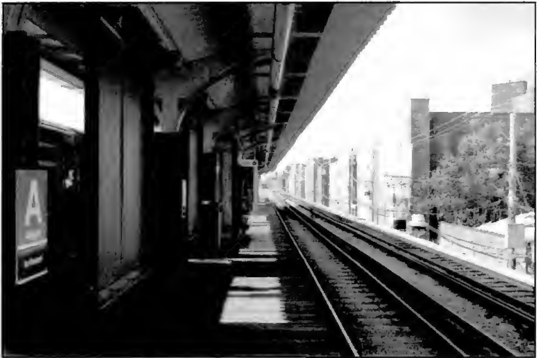
West Argyle Street elevated platform (1922)
